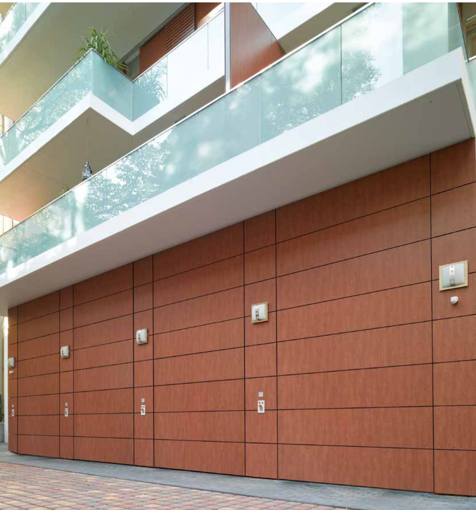
On-site cladding with laminated timber boards
