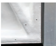
The "flowcoat" provides a smoother finish as shown on the bottom corner detail illustrated left
