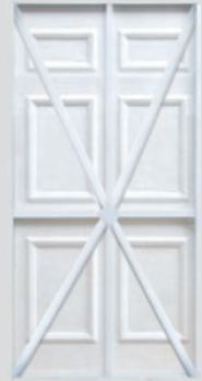
The neat inner face and steel bracings
