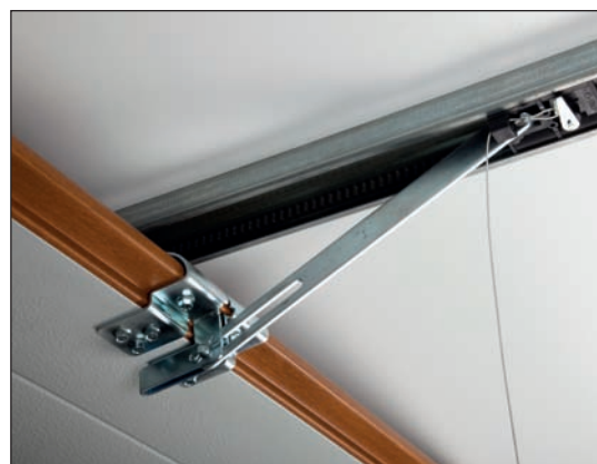
General arrangement of drawbar connector cleat (may vary according to headroom).
